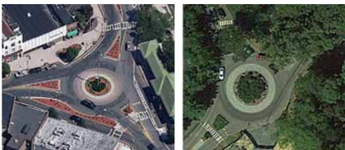
Figure 2a. Sample Study Sites Example of Roundabouts
