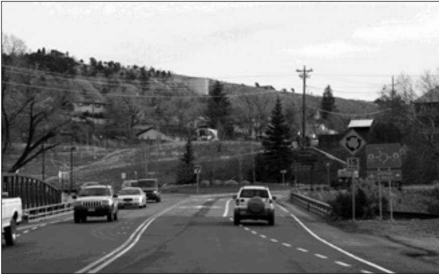
Figure 5. Capacity improvements along Eby Creek Road completed October 2008. Looking south at the US 6 roundabout with added approach lane to accommodate heavy right-turn movement.
