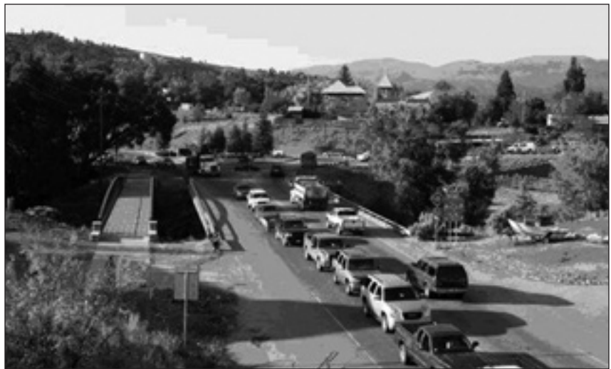
4a. Looking south toward roundabout.
