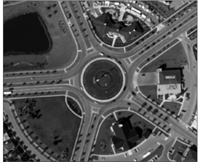
Figure 2. The first modern roundabout appeared on Calgary's landscape in 1998.
