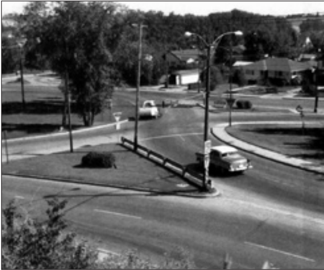
Figure 1. The first use of a circular intersection in Calgary, Canada.
