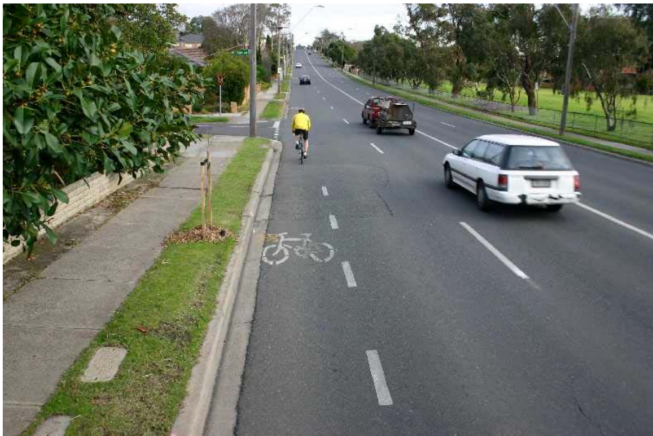
Figure 4 – Wide Kerbside Lane Marking With Bicycle Symbol And Short Longitudinal Line
