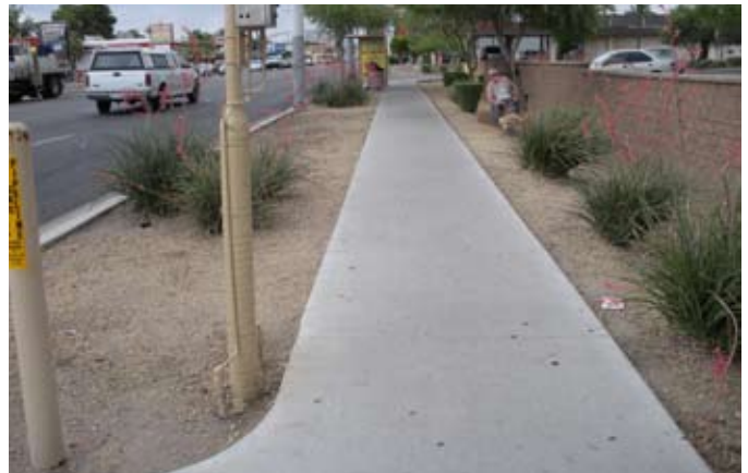
Notice the extensive landscaping and buffering adjacent to the sidewalk; this adds to the environment comfort for walking.
