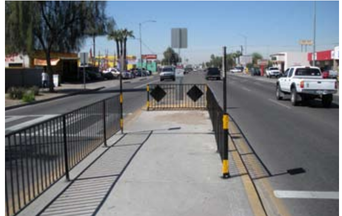
Example of a two-stage crosswalk.
