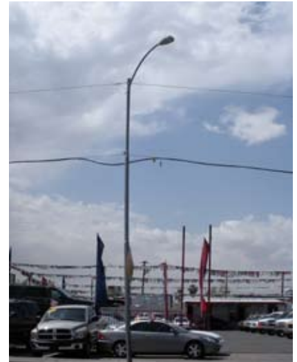
Light pole turned the wrong way.
