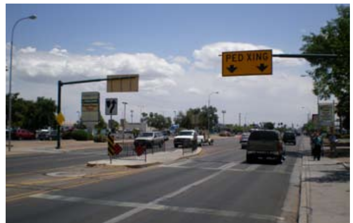
Overhead sign designating the crosswalk location.
