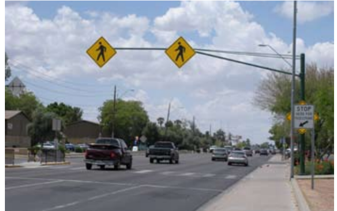
Overhead and side-mounted signs designating the crosswalk location.
