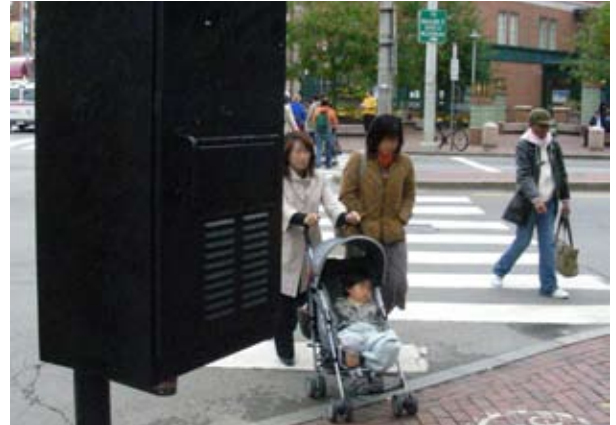
Pole-mounted cabinet on southwest corner that could be a hazard to visually impaired pedestrians.
